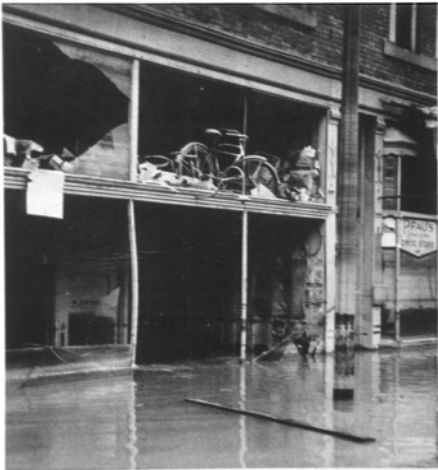
Pfau's Drug Store at 329 Spring Street in Jeffersonville — Water going down.
